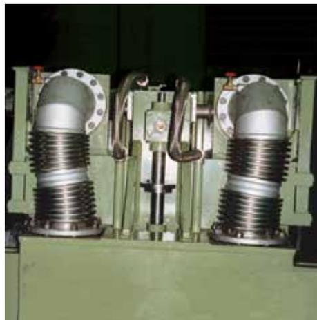
UM type expansion joints installed on an engine.
