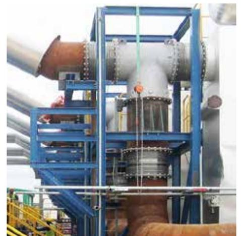
UM type expansion joints installed at a flue gas exhaust system at a power plant.
