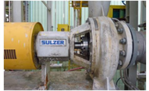
An EagleBurgmann **MA291/60** type single cartridge seal is installed in a Sulzer APP pump at an Indonesian paper mill. The medium to be sealed is pulp with a solids content of 5.5 %. Operating conditions:  $p = 4 \text{ bar (58 PSI)}$ ,  $t = 60 \text{ }^\circ\text{C (140 }^\circ\text{F)}$ ,  $n = 1,430 \text{ min}^{-1}$ .
