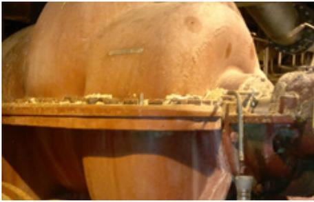
At the UPM Pietarsaari paper mill in Finland, a feed pump for pressure screens is sealed by an EagleBurgmann **LP-Q-SA2-DZXX70/160**. Installed since 1988, overhauled in 2000, it operates reliably up to today. Operating conditions:  $p = 2 \dots 3 \text{ bar}$  (29 ... 44 PSI),  $t = 60 \text{ °C} \dots 70 \text{ °C}$  (140 °F ... 158 °F),  $n = 750 \text{ min}^{-1}$ .
