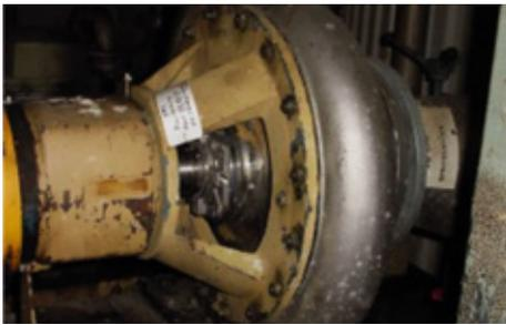
At Stora Enso Kvarnsveden, Sweden, several pumps of the paper machines are sealed with EagleBurgmann **MA251**. Medium: pulp with a solids content up to 1.5 %. Operating conditions:  $p = 2 \text{ bar}$  (29 PSI),  $t = 30 \text{ °C} \dots 40 \text{ °C}$  (86 °F ... 104 °F),  $n = 1,490 \text{ min}^{-1}$ .
