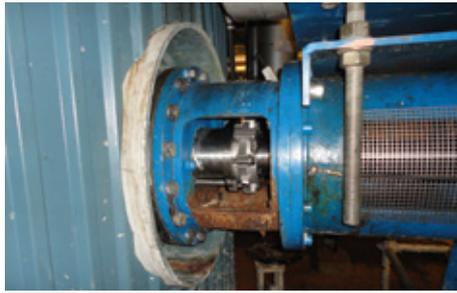
After retrofitting at Stora Enso in Sweden, two fully split EagleBurgmann **Splitex** type mechanical seals operate successfully in a mixer with bottom entry and a chest agitator with side entry. Here, pulp having a solids content of over 11 % is sealed. Operating conditions:  $p = 10.3 \text{ bar (149 PSI)}$ ,  $t = 180 \text{ }^\circ\text{C (356 }^\circ\text{F)}$ ,  $n = 15 \text{ min}^{-1}$ .
