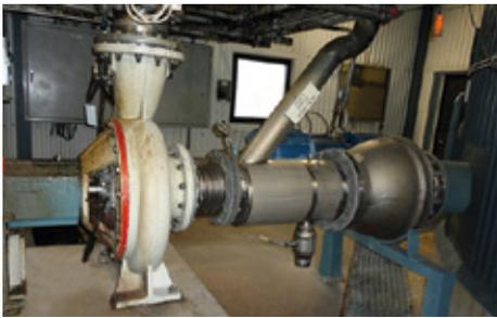
In the pulp production at Stora Enso Skutskär in Sweden, a Sulzer APP Ahlstar pulp pump transports the pulp with black liquor to the washing and bleaching processes. The pump is equipped with an EagleBurgmann **Cartex-DN** with a connected **BestFlow** pressure regulating valve for the optimum supply of buffer water to the seal. Operating conditions:  $p = \text{max. } 4.5 \text{ bar (65.3 PSI)}$ ,  $t = 66 \text{ }^\circ\text{C (151 }^\circ\text{F)}$ ,  $n = 956 \text{ min}^{-1}$ .
