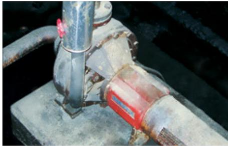
At the UPM Pietarsaari pulp mill in Finland, a Sulzer APP 23 pump is sealed with an EagleBurgmann **Mtex-TN**. This cartridge version of the metal bellows seal is particularly suitable for highly viscous media at low temperatures. Operating conditions:  $p = 1 \text{ bar (15 PSI)}$ ,  $t = 120 \text{ }^\circ\text{C (248 }^\circ\text{F)}$ ,  $n = 1,500 \text{ min}^{-1}$ . Medium: Tall oil.
