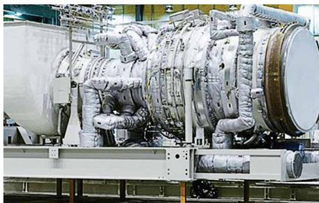
A **fabric expansion joint** manufactured by EagleBurgmann Expansion Joints Solutions installed in a Siemens SGT 800 gas turbine. Operating conditions:  $p = -9.8 \dots +14 \text{ mbar}$  (-142 ... 203 PSI),  $t = 620 \text{ }^\circ\text{C}$  (1,148 °F), gas flow rate: 40 m/s, axial displacement -34 mm, lateral displacement +4 mm.
