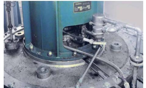
EagleBurgmann **HGH210/225-E1** are installed in the main cooling water pump at the KNG power plant in Rostock. Operating conditions:  $p = 2.25 \text{ bar}$  (23.63 PSI);  $t = 25 \text{ }^\circ\text{C}$  (77 °F);  $n = 490 \text{ min}^{-1}$ ; medium: brackish water with sand.
