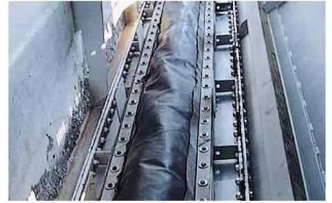
**Fluastal** expansion joints (9 x 5 m) made of special fabric are installed in a flue gas duct at the EGAT Wang Noi power plant in Thailand. Operating conditions:  $p = 0.074 \text{ bar}$  (1.07 PSI);  $t = 580 \text{ °C}$  (1,076 °F).
