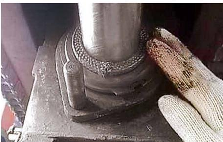
At the PT.Ipmomi coal-fired power plant in Indonesia, sealing for high temperature exhaust gas which contains fly ash and steam is needed on a soot blower. **Isartherm 6011A** and **Isartherm-Flex 6050** compression packings help to maintain safe and reliable operation. Operating conditions:  $p = 40 \text{ bar}$  (580 PSI);  $t = 400 \text{ }^\circ\text{C}$  (752 °F).
