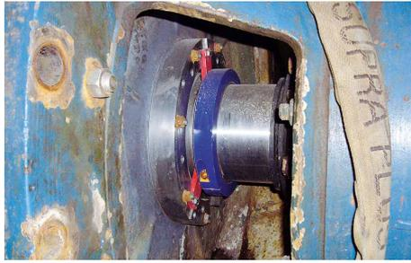
A suspension pump is used to circulate abrasive milk of lime at the RWE power plant in Frimmersdorf, Germany, sealed with an EagleBurgmann **HR325/270-G11-E6** mechanical seal. Operating conditions:  $p = 3 \dots 4.5 \text{ bar}$  (44 ... 65 PSI);  $t = 50 \text{ }^\circ\text{C}$  (122 °F);  $n = 890 \text{ min}^{-1}$ .
