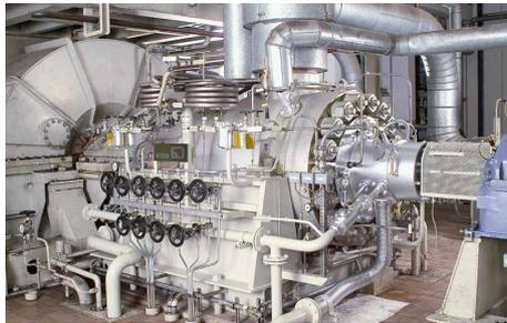
A **SHV1/200-E1** mechanical seal is installed in a KSB CHTA140 feedwater pump at the ENBW power plant in Heilbronn, Germany. Operating conditions:  $p = 30 \text{ bar}$  (435 PSI);  $t = 180 \text{ }^\circ\text{C}$  (356 °F);  $n = 5,100 \text{ min}^{-1}$ .
