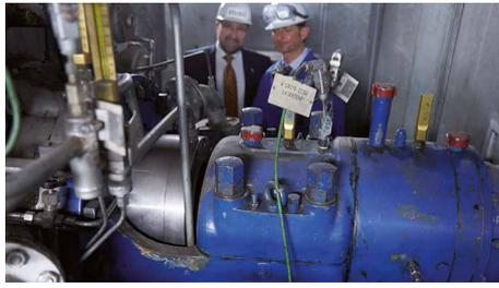
The EagleBurgmann **DF-SAFI4/188** diamond-coated mechanical seal runs in the boiler feed pump of the black coal power station in Voerde, Germany, to the complete satisfaction of the operator. Operating conditions:  $p = 21 \text{ bar (305 PSI)}$ ;  $t = 158 \text{ }^\circ\text{C (316 }^\circ\text{F)}$ ;  $n = 5.100 \text{ min}^{-1}$ .
