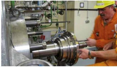
In a German power station, the shafts of the main feed pumps are sealed with EagleBurgmann type **DF-SAF1/165** mechanical seals with DiamondFace coating.
